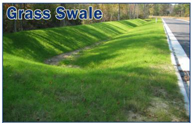
A narrow trench that's either planted or kept as grass. Great for along roads to capture runoff, sending it to either the ground or filtering it before it gets to a lake or wetland.
