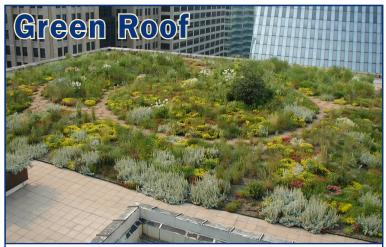
A roofftop garden with layers of soil and gravel beneath it to store water for dry periods. Excess is piped off of roof.
