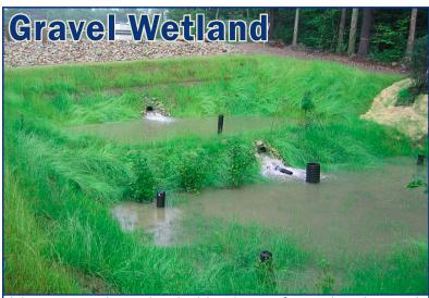
A human-made wetland with a layer of gravel underneath it. Great for sandy areas or low spots close to the water table (groundwater). Plants and soil work together to absorb and infiltrate water.
