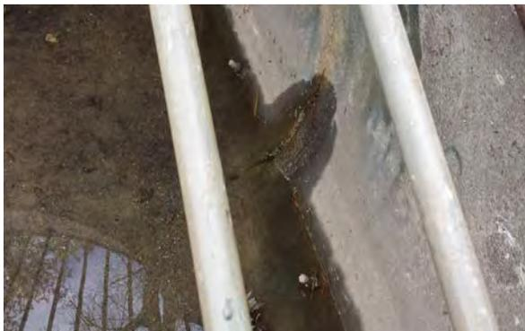
Groundwater infiltration into storm drain at Whitaker Monitoring Site outfall
