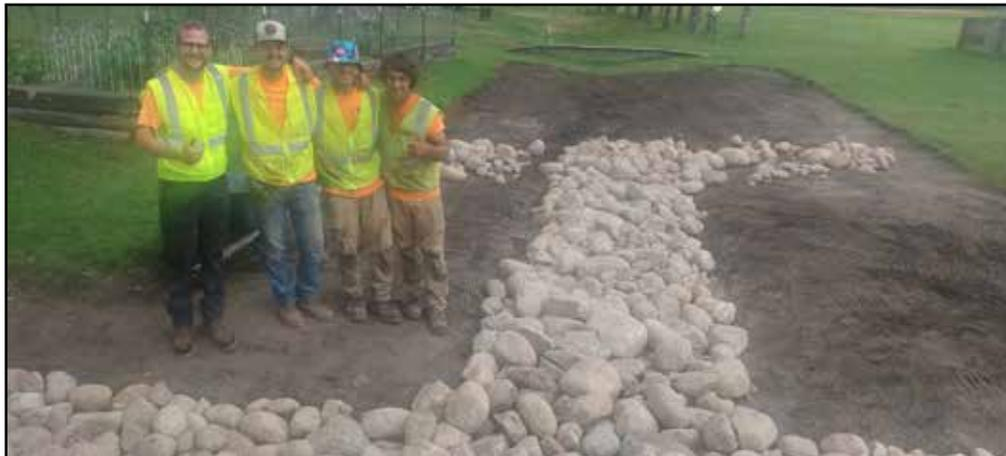
Top: The newly constructed and newly planted bioswale looking southwest towards the Basswood wetland. The culvert beneath the walking path was pre-existing and the bioswale was built around it.
