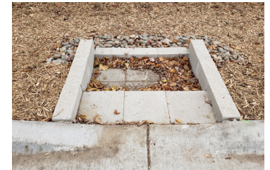
Above: A completed curb cut raingarden in the City of White Bear Lake awaiting spring 2025 native plantings.
