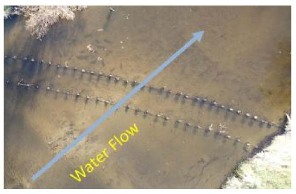
Two strips of low voltage electrodes on the bottom substrate compose the barrier on Rice Creek.
