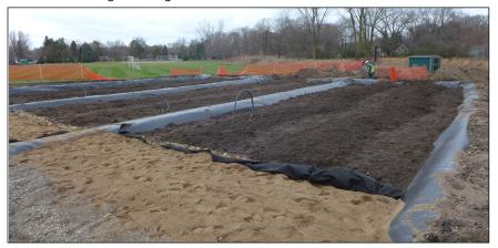
Three wetland cells are filled with sorptive material and ready for Spring planting.
