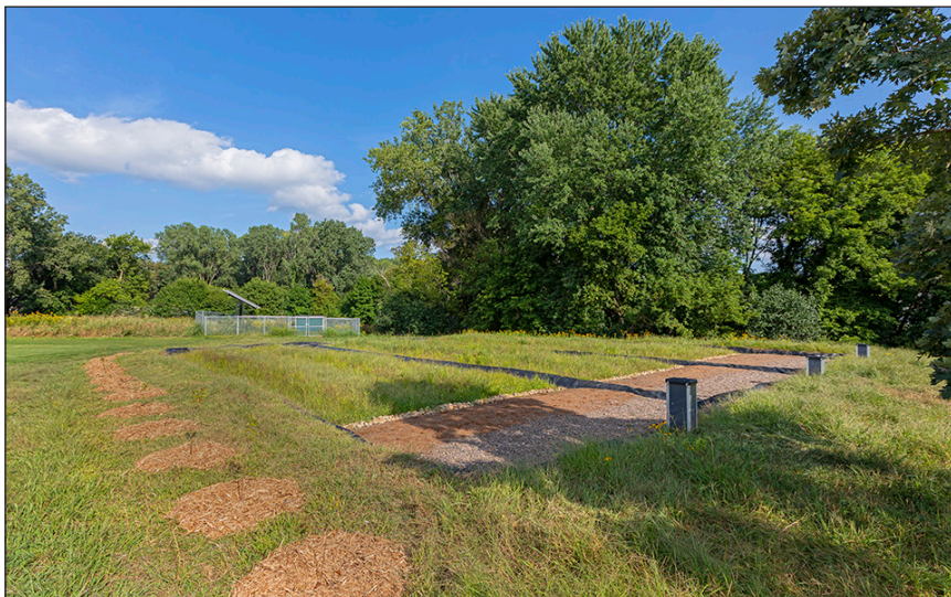
Three wetland cells are filled with sorptive material .
