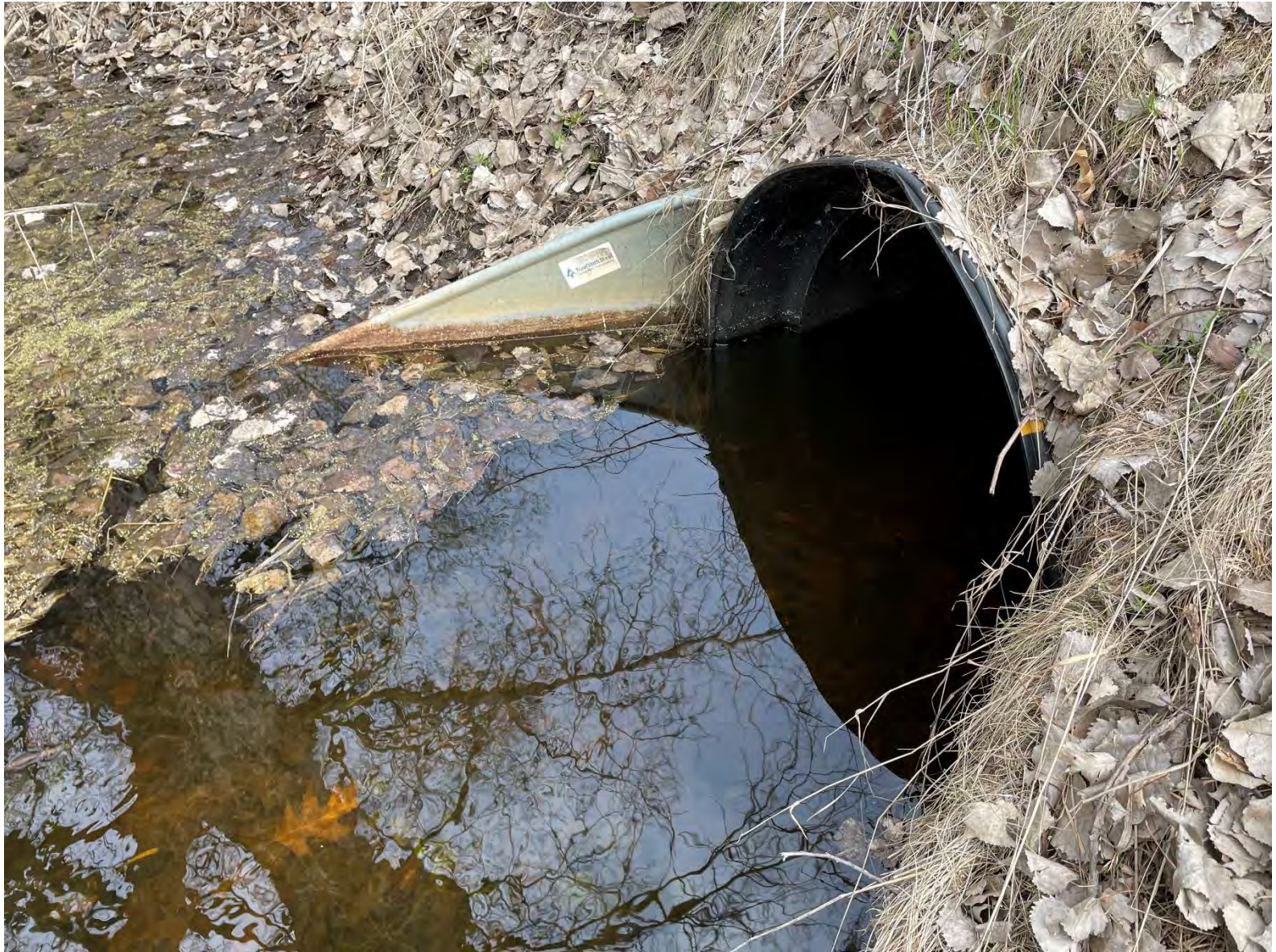
22 - Culvert E Downstream End
