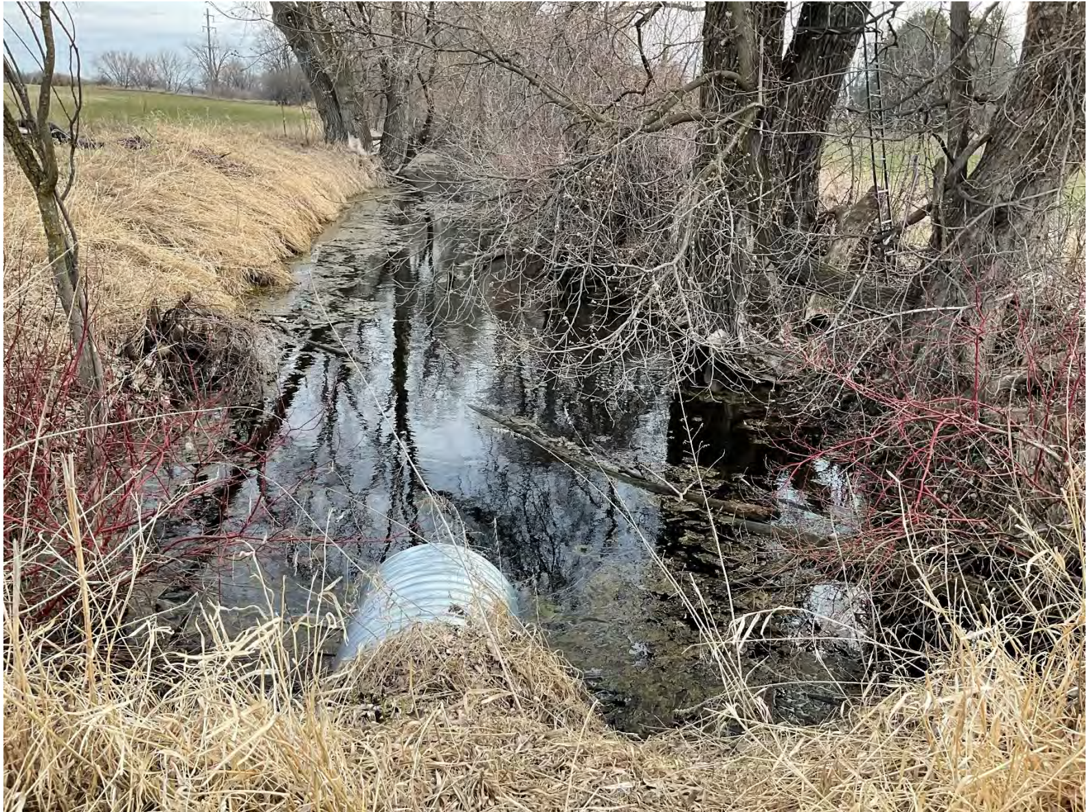
30 – Culvert F Upstream Channel
