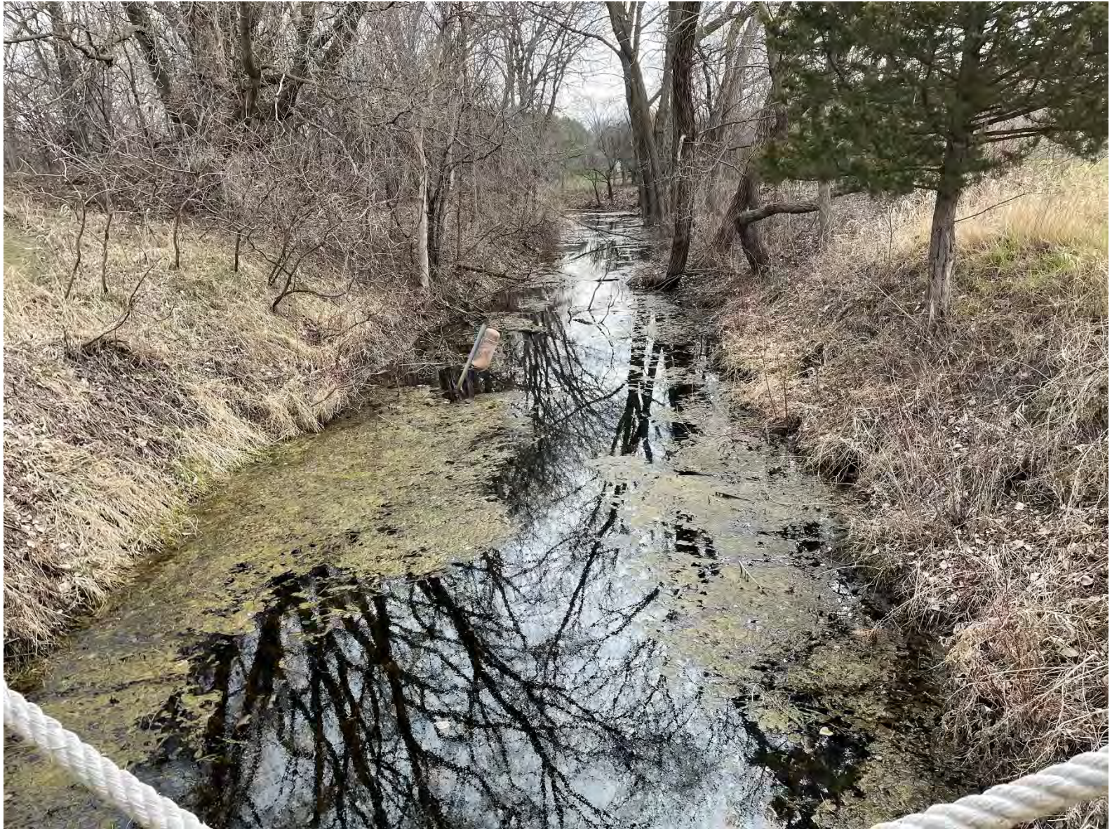
25 - 6433 20 th Ave Bridge Upstream Channel
