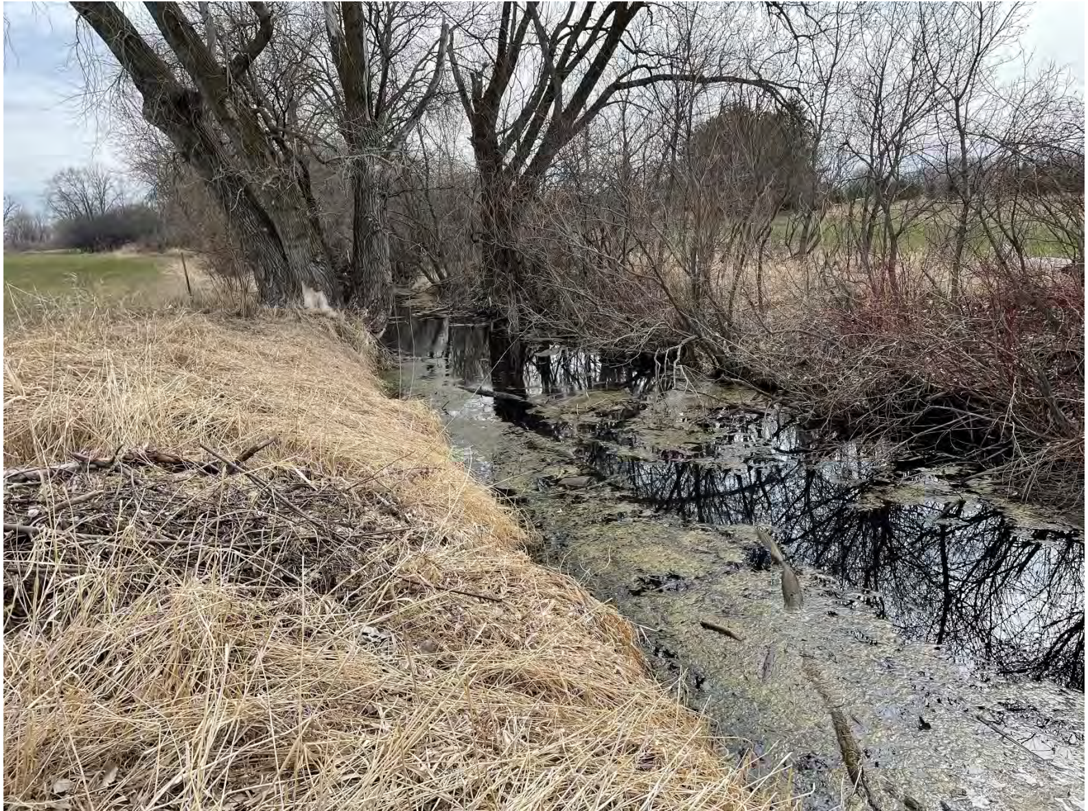
29 – Culvert F Upstream Channel
