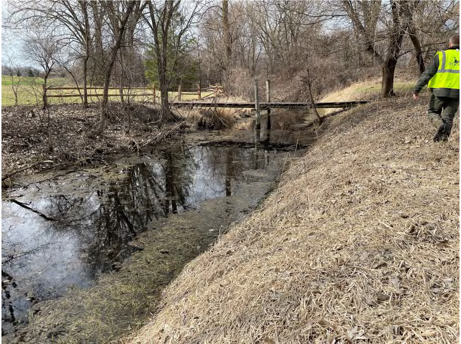
19 – Channel in 6443 20 th Ave Property
