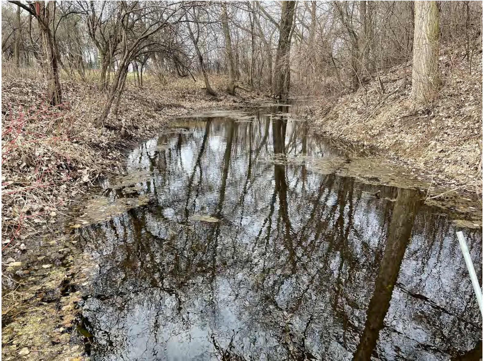
24 - Culvert E Downstream Channel
