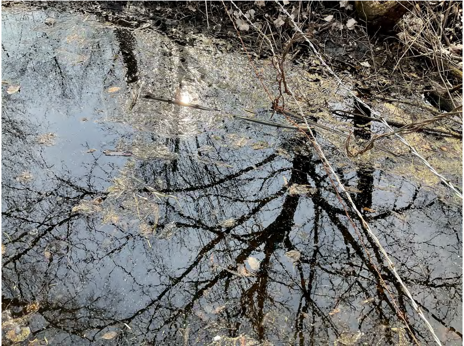
15 – Narrowing of Channel Near Side Ditch
