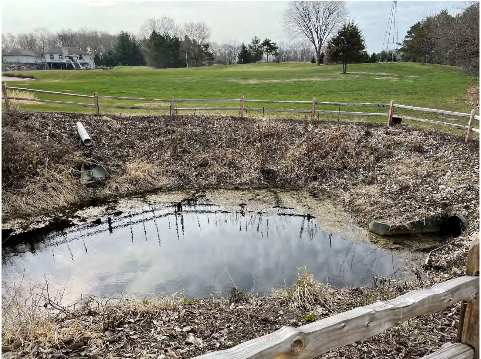
21 - Culvert E Upstream Pool
