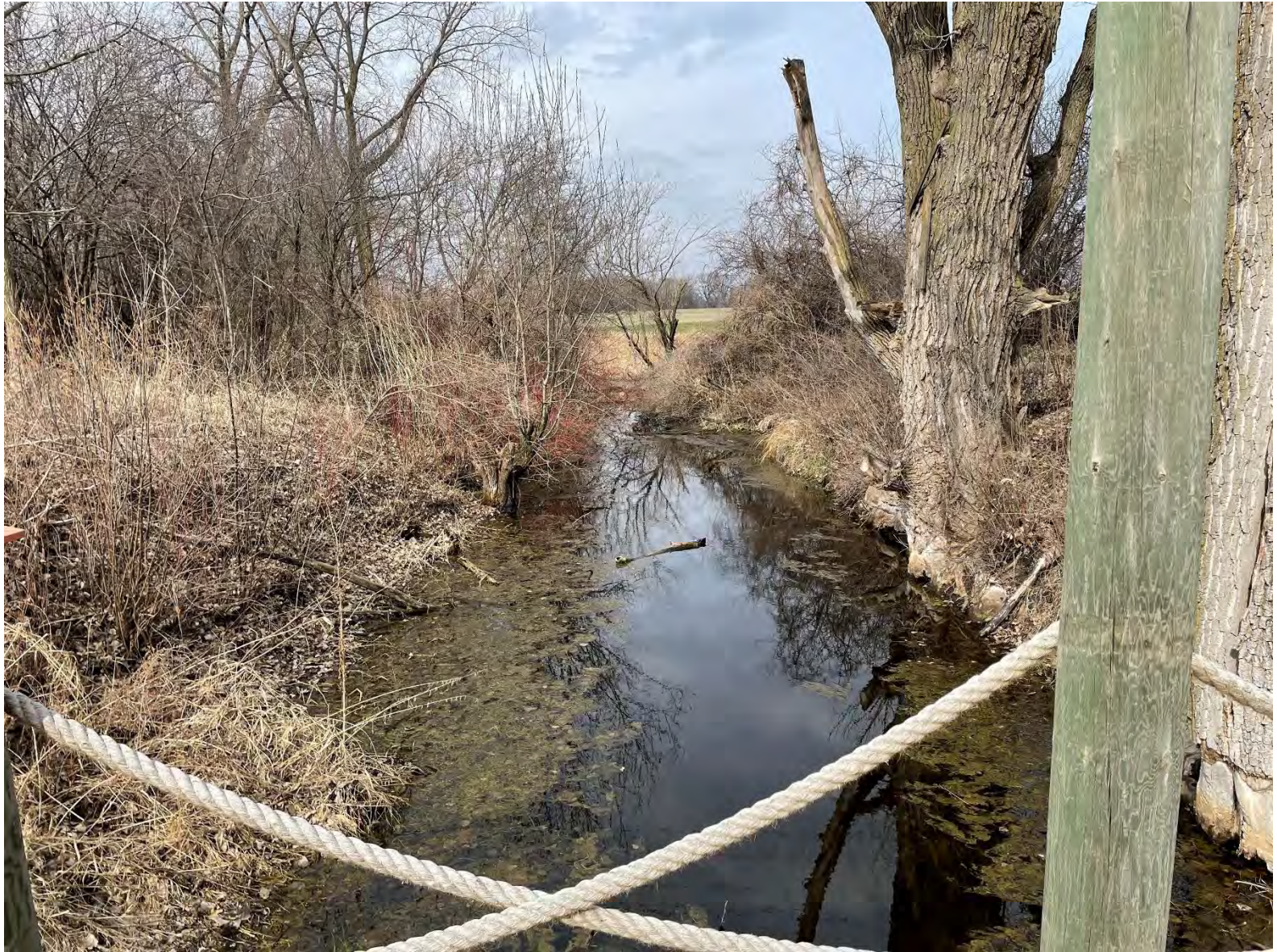
26 - 6433 20 th Ave Bridge Downstream Channel
