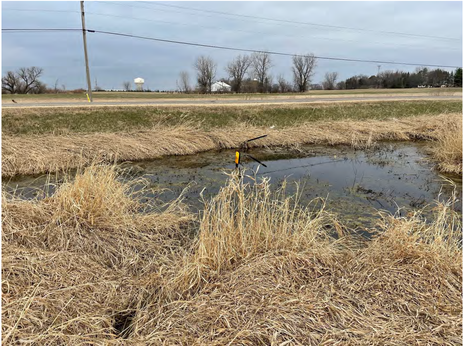
1 – Culvert C Upstream
