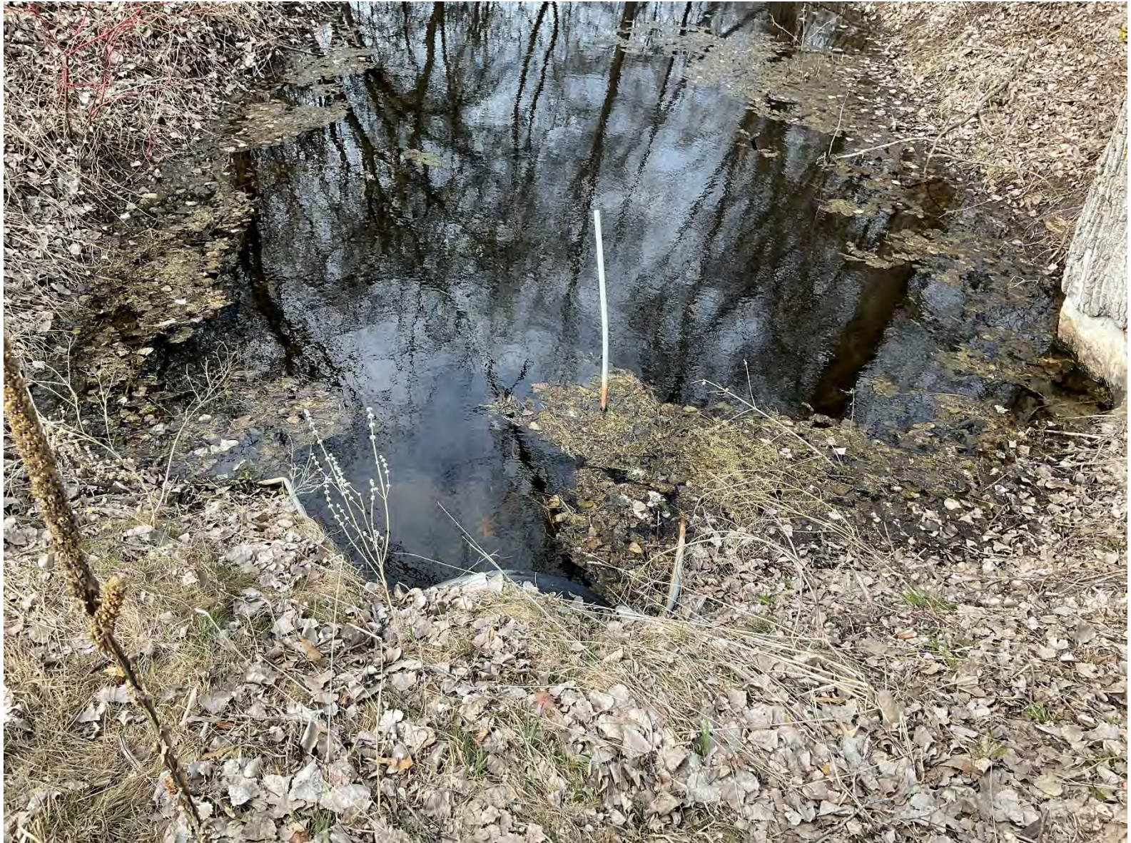
23 – Culvert E Downstream End
