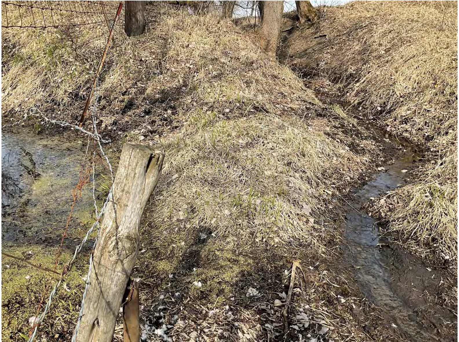
16 – Side Ditch Delta
