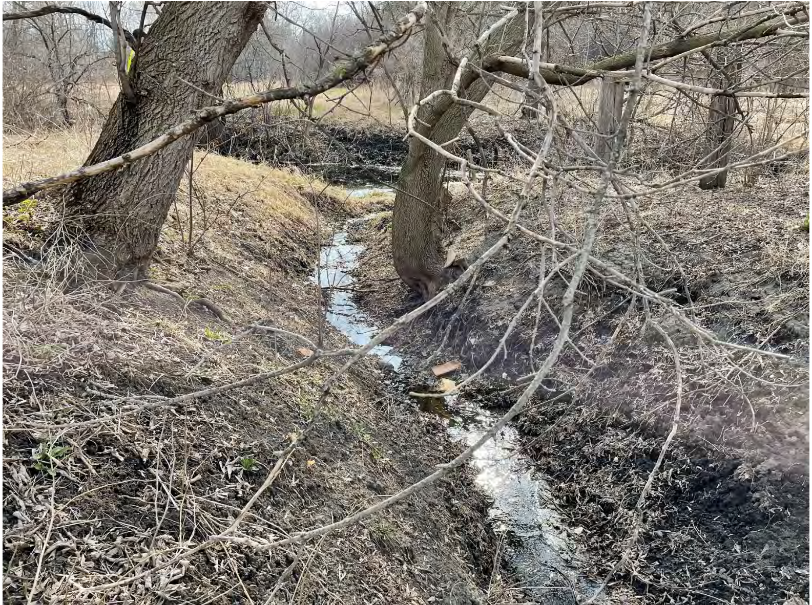
18 – Looking East Down Tributary Side Ditch
