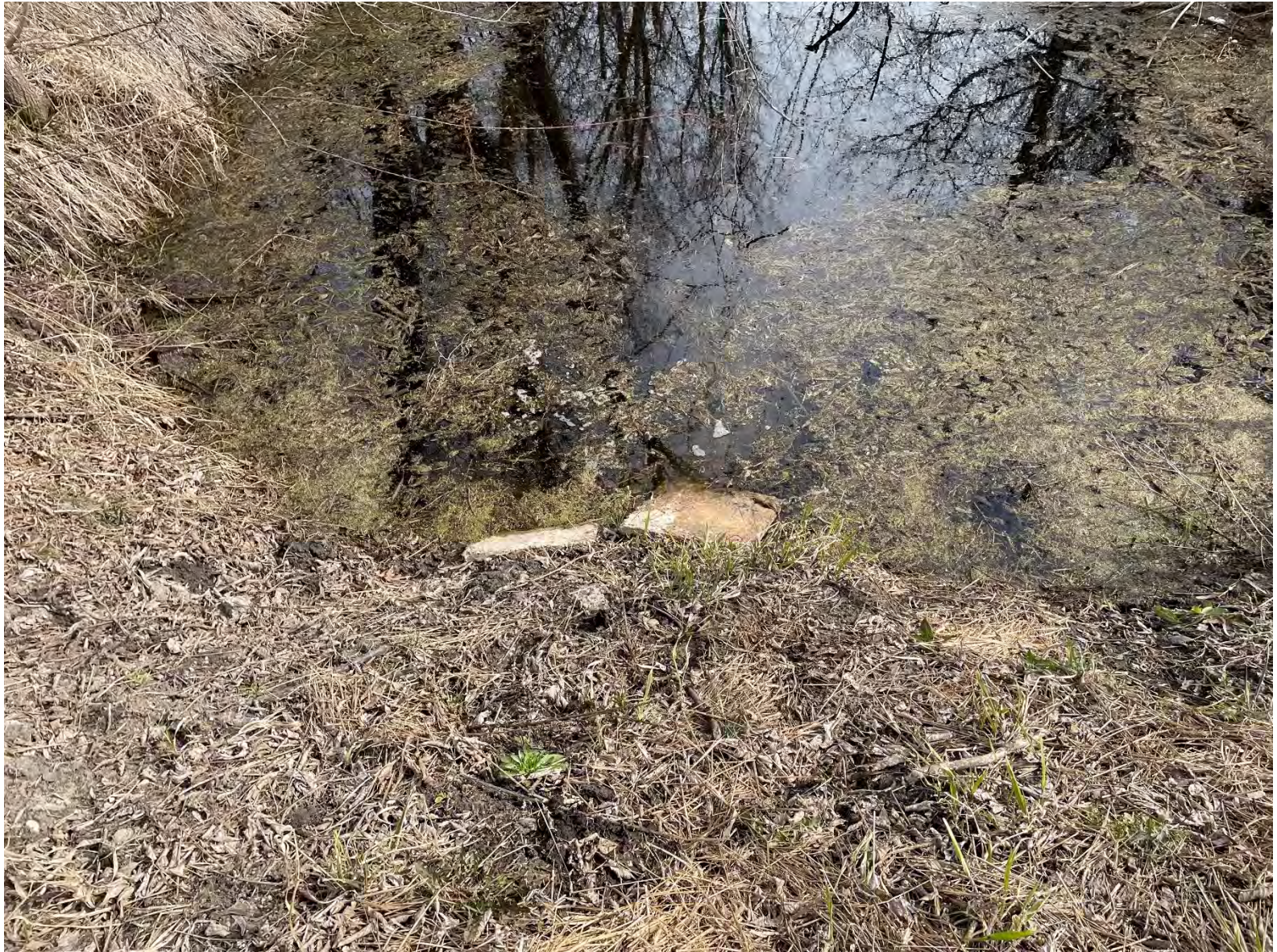
9 –Upstream End of Culvert D
