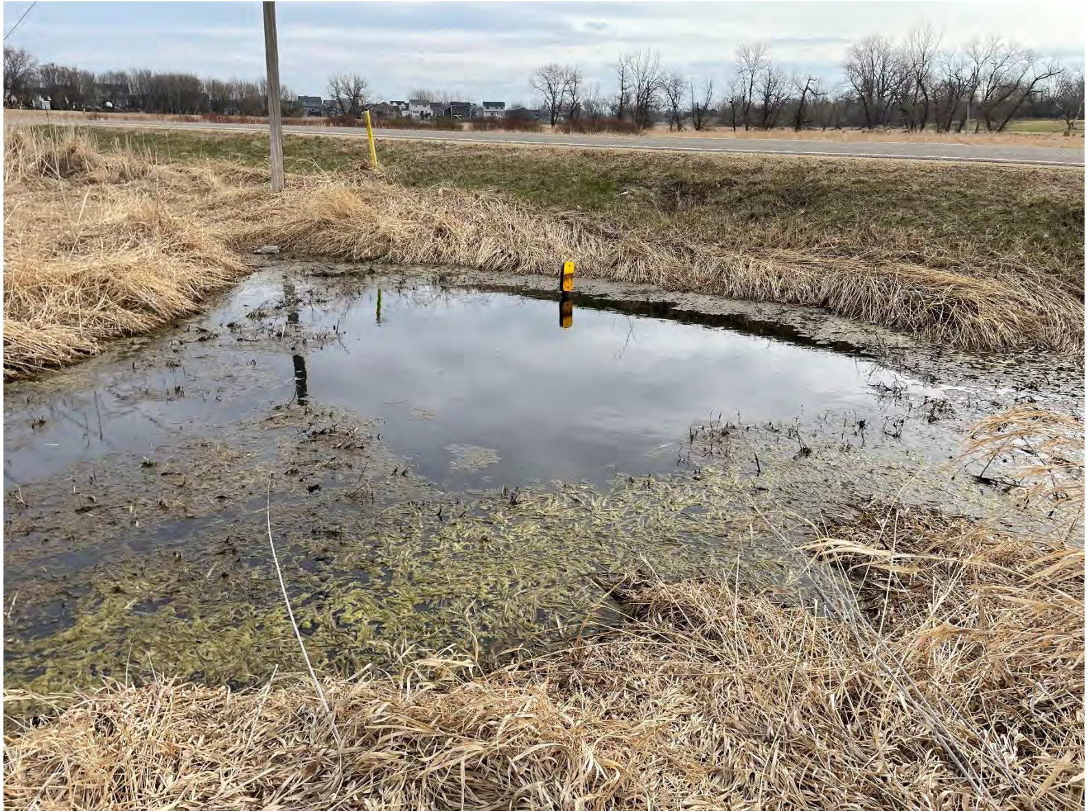
5 –Culvert C Downstream
