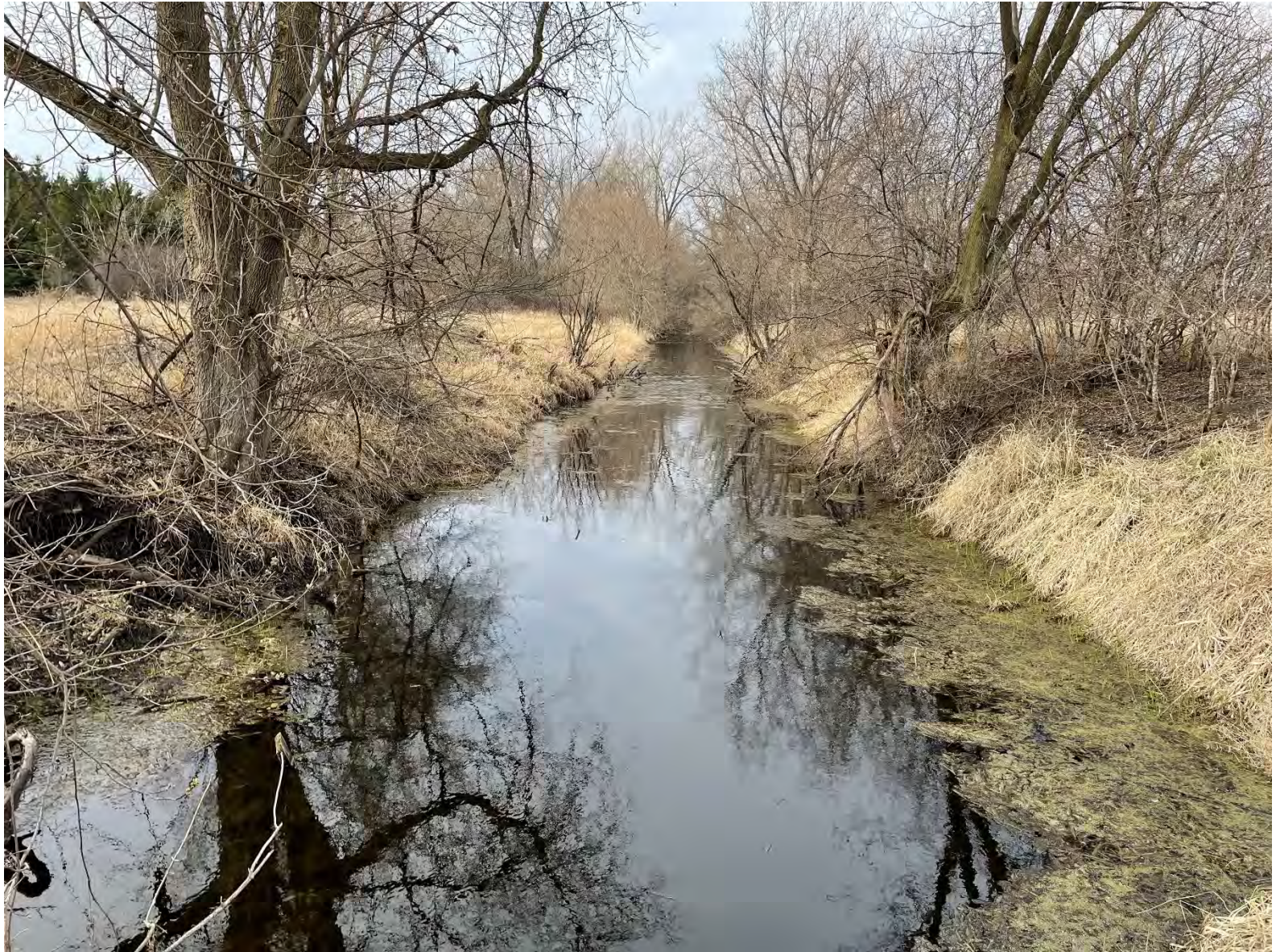
11 – Channel Downstream of Culvert D
