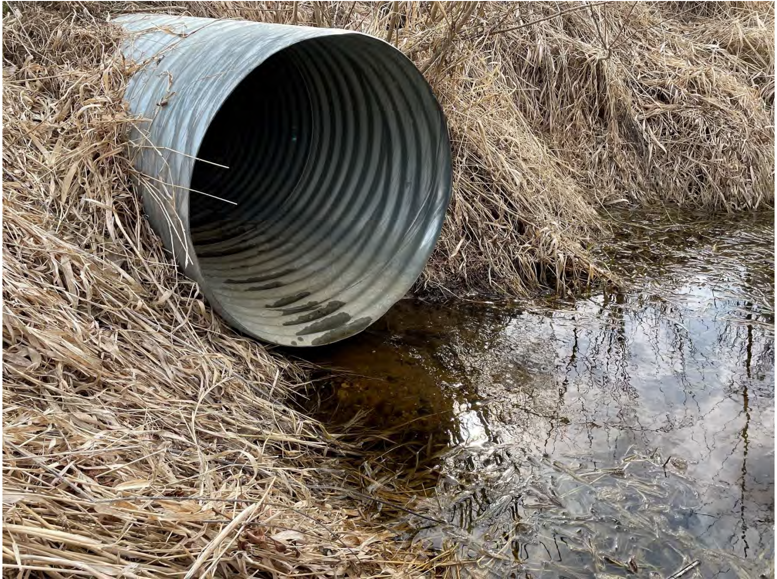
31 – Culvert F Downstream End
