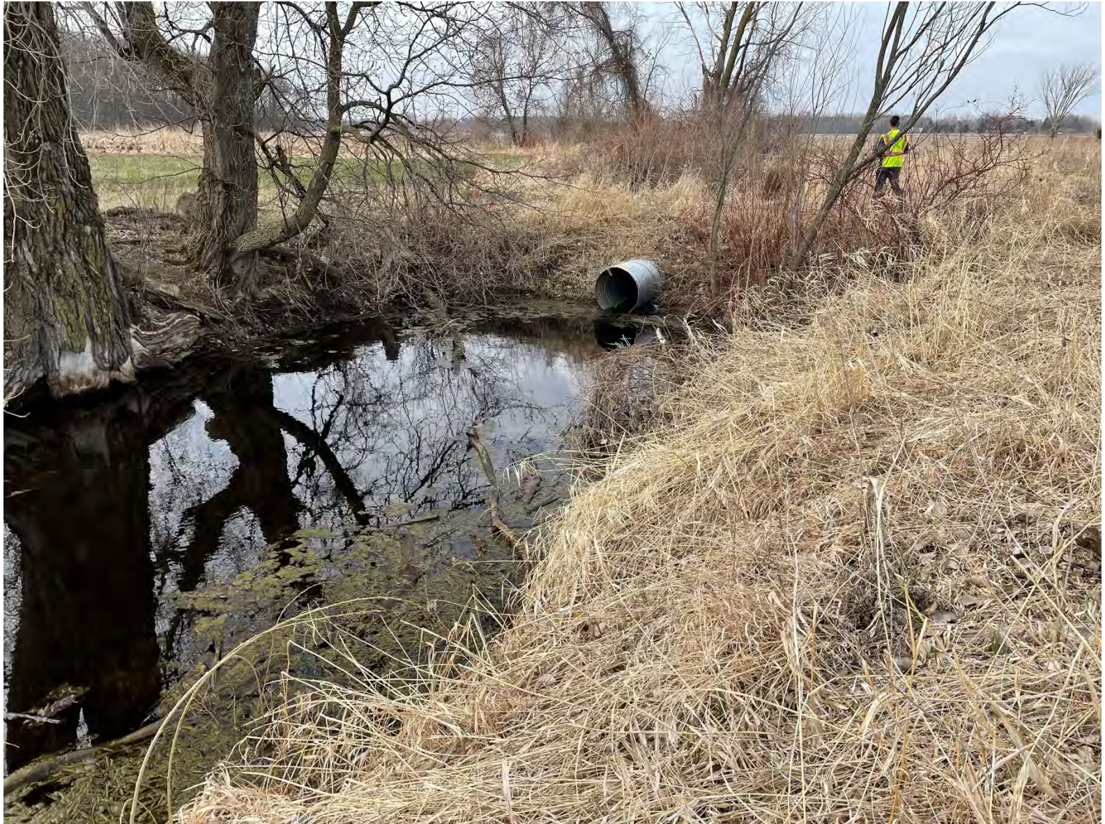
28 – Culvert F Upstream Pool
