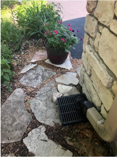
Drain collection box
