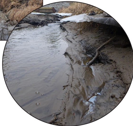
Lambert Creek dredging: Construction (above) and post-dredging creek level (right), evidenced by former water level ice shelf and new water level at creek bottom.
