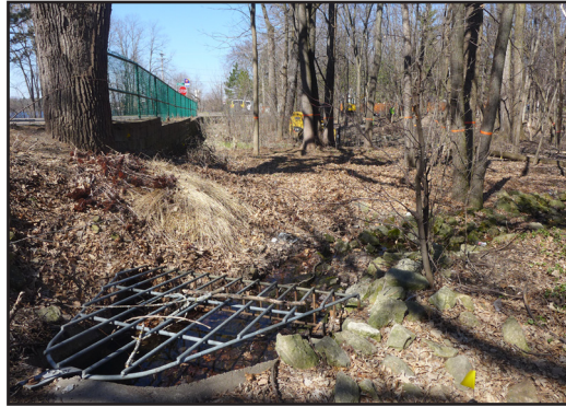
Above: Pre-construction, the stormwater outfall draining untreated stormwater into the wetland and Birch Lake. Right: Construction, filter completion, and the complete filter fresh after a rain event in July, 2020.
