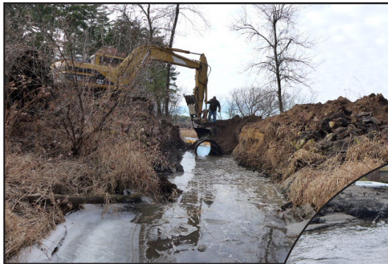
Lambert Creek dredging: Construction (above) and post-dredging creek level (right), evidenced by former water level ice shelf and new water level at creek bottom.
