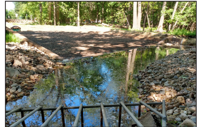
Above: Pre-construction, the stormwater outfall draining untreated stormwater into the wetland and Birch Lake. Right: Construction, filter completion, and the complete filter fresh after a rain event in July, 2020.
