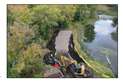
Above: The Whitaker Pond Biochar Filter pictured during construction in October 2022.
