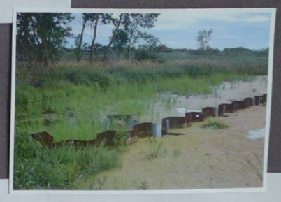
New metal sheet pilings were installed in 2012 to replace the original plastic pilings that were showing signs of failure; new pilings were crucial to prevent a blowout and downstream damage to property and projects
