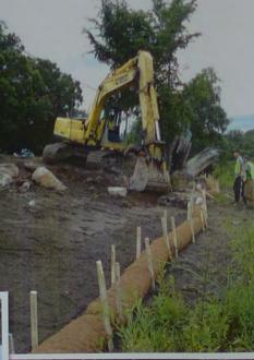
♦ The project consisted of clearing and replanting with deep-rooted native vegetation that withholds soil for a stable shoreline to withstand erosion
