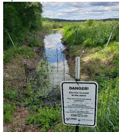
Electrified barrier on southern wetland at modified culvert (2020)
