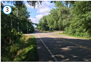
East Vadnais Lake Subwatershed Outfall Location to be Rebuilt with the Edgerton Road Drainage Improvements Plan.
