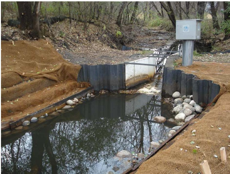
The flumes were installed on Koehler Road and County Road F in Vadnais Heights, and Oakmede Lane in White Bear Township. These sites allow for safe and reliable sampling locations, as well as locations to measure streamflow and volume.
