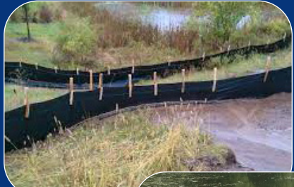
Silt fences and curtains
