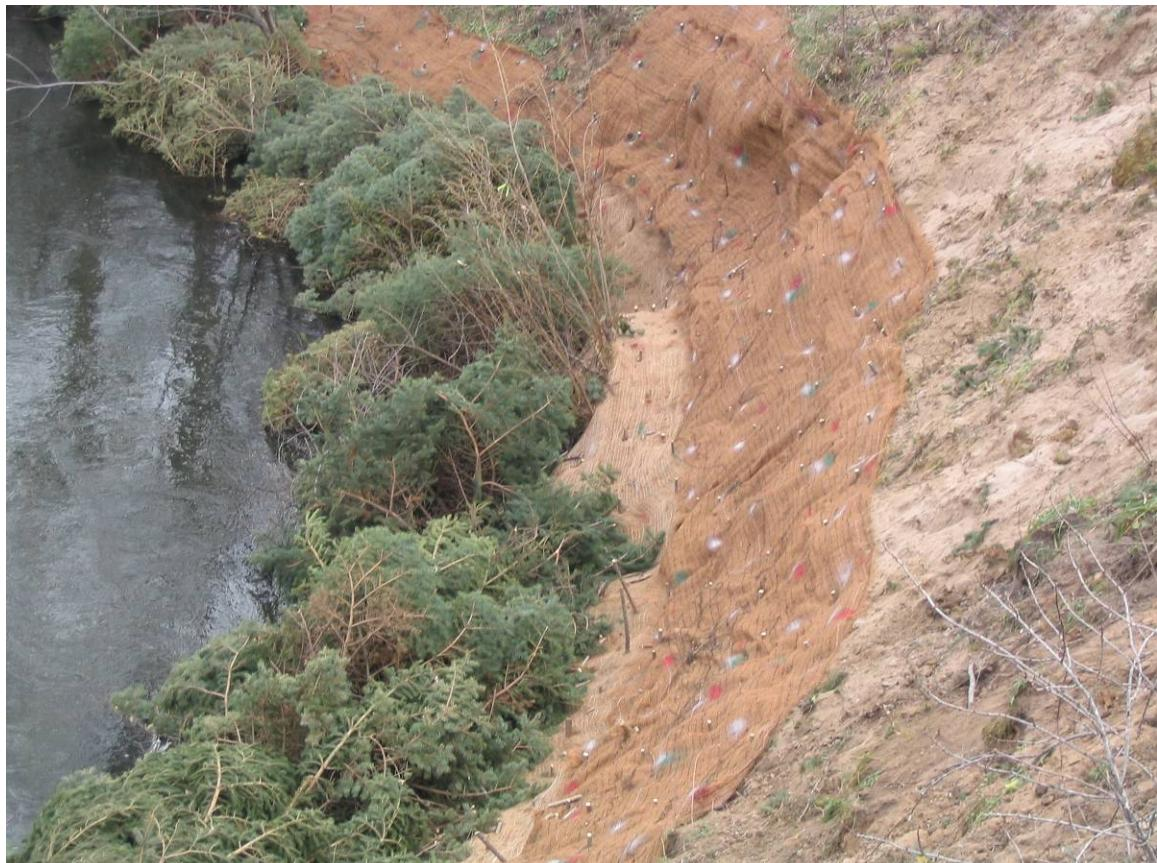
**Figure 54. Use of trees for revetment along toe of eroding slope on Vermillion River, Hastings, MN.**
