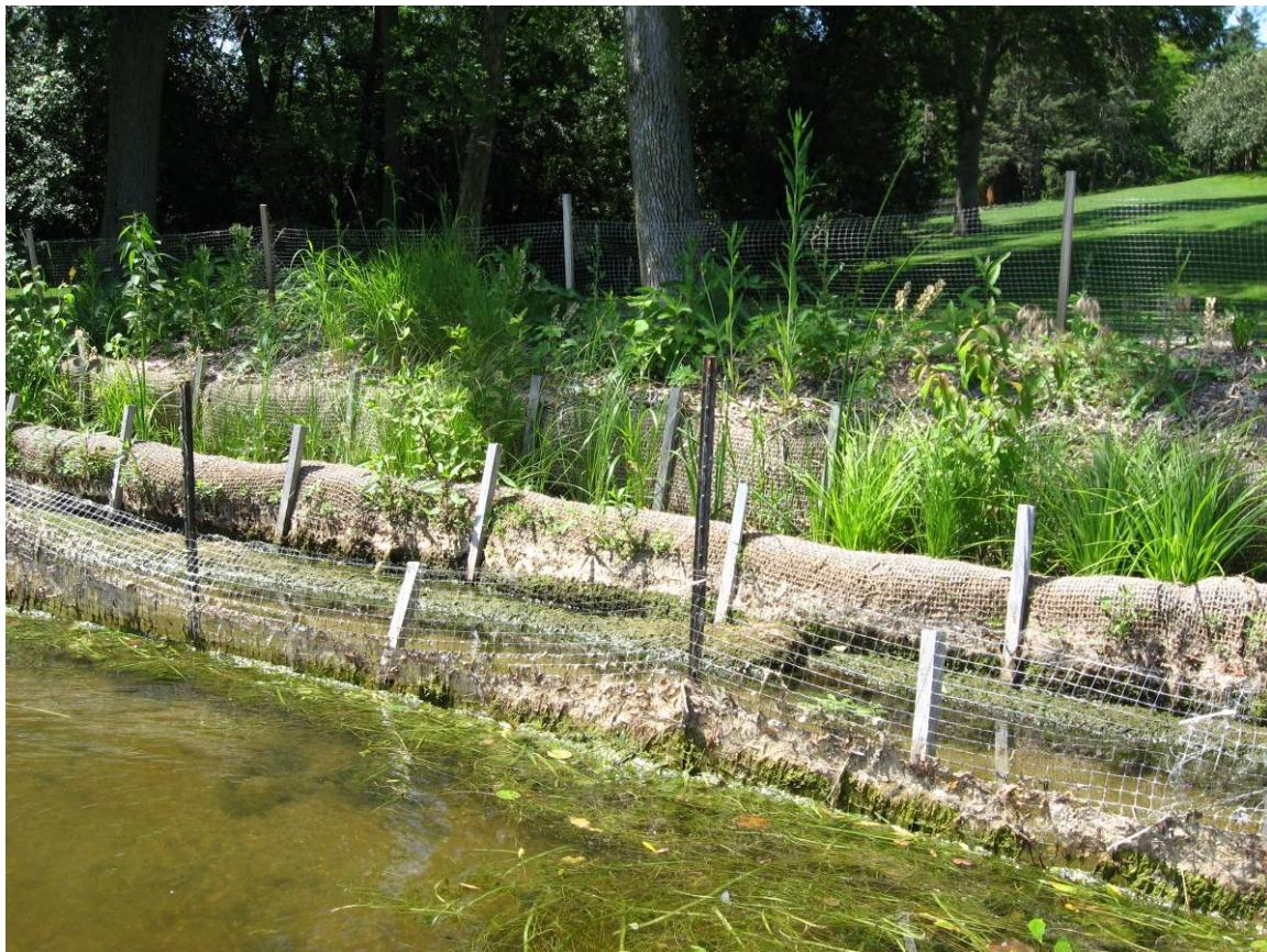
**Figure 48. Use of Bio-D-Blocks at 16 Evergreen Road lakeshore site.**
