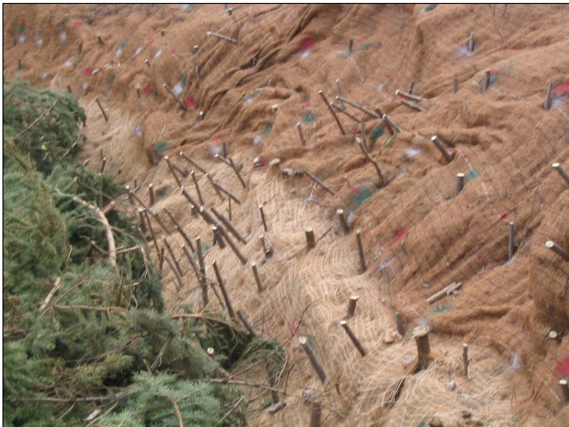
**Figure 38. Live willow stakes just after installation on a shoreline.**
