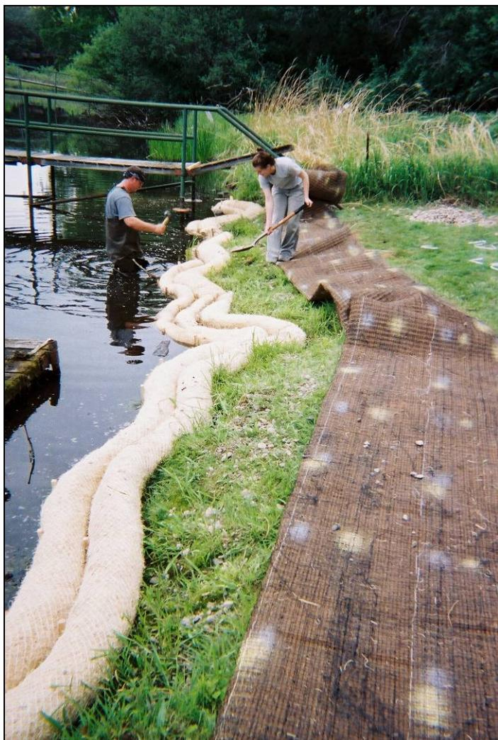
**Figure 47. Use of wood-fiber biologs for shoreline restoration.**
