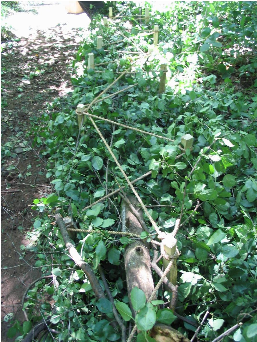
**Figure 53. Use of Brush Mattress at Silver Creek streamline restoration in Stillwater, MN.**
