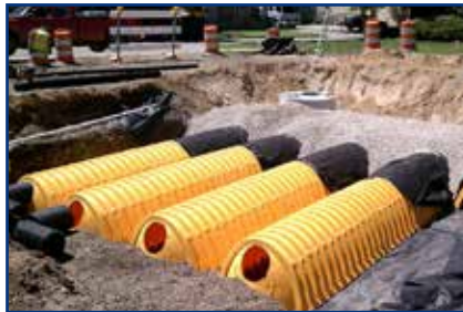
Underground retention basin
