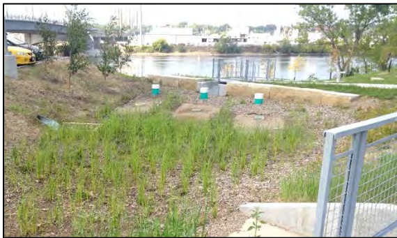
One rain garden includes the Filter Media Test Lab. This feature directs runoff through three buried pipes containing different filtration media: clean sand, iron-enhanced sand, and spent lime.
