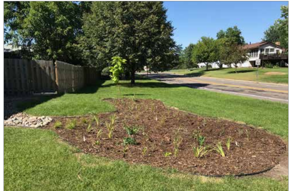
A 2018 raingarden install in Vadnais Heights
