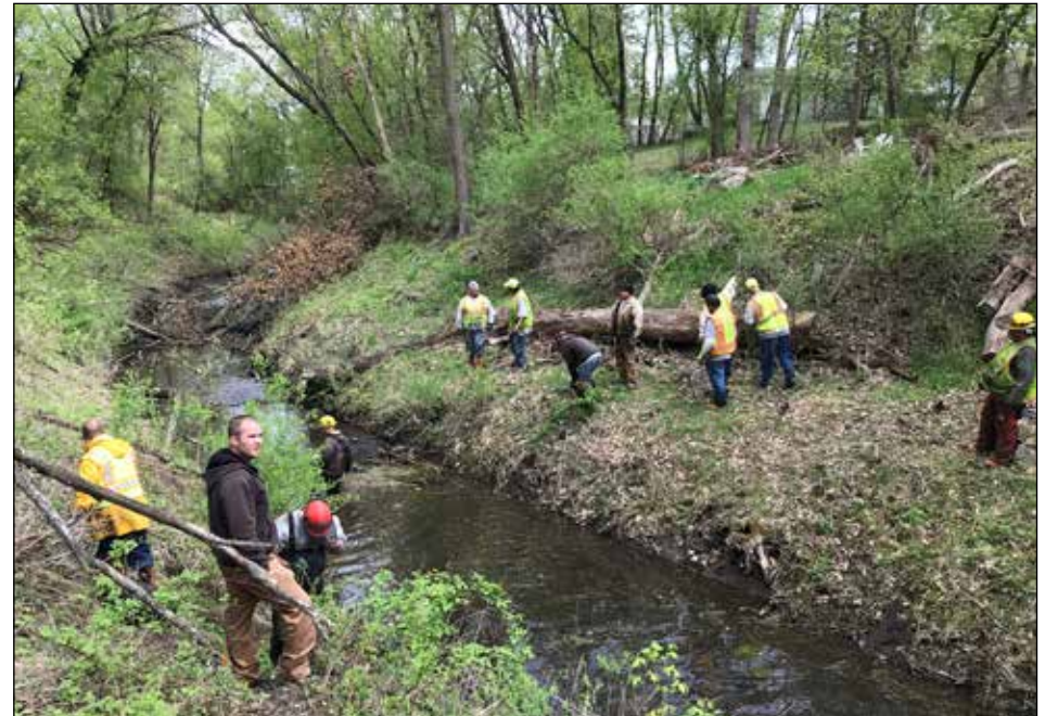
ICWC clearing debris in Lambert Creek
