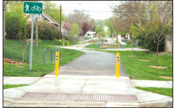
The completed greenway benefits residents and the traveling public by reducing flooding, reducing impervious surfaces, improving water quality, and enhancing public space.
