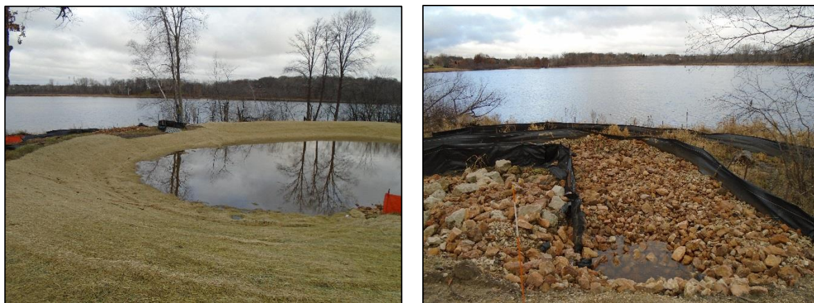
Figure 10. Location for proposed iron enriched sand filter. Filter can take form of a bench in the Charley Lake Preserve stormpond (left) or as an installation in the rip-rap at the outlet (right).
