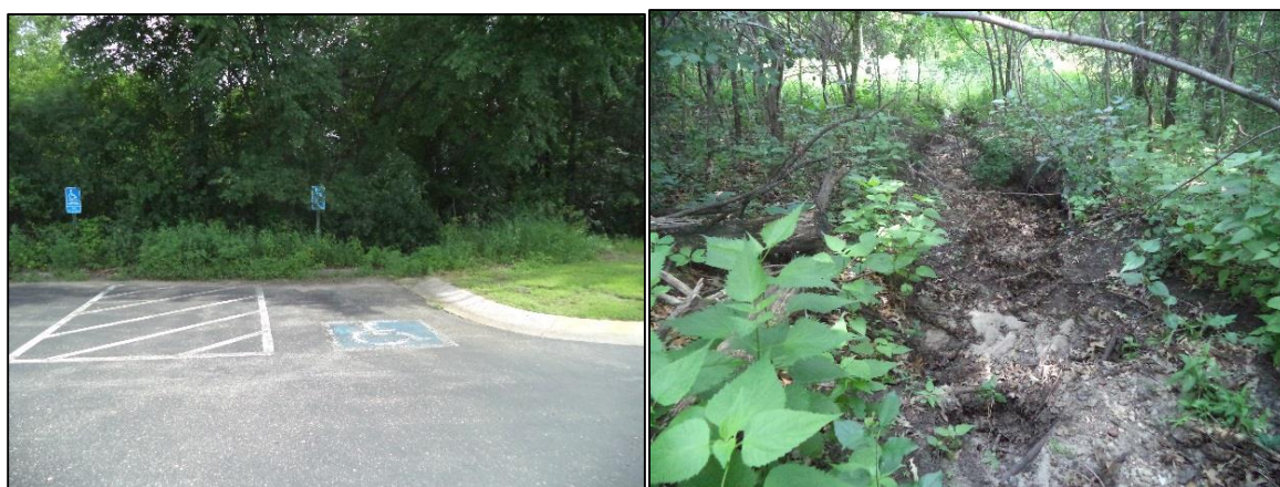
Figure 9. Location for retrofit 7 (left). Proposed removal of 4 parking lots and installation of rain garden to treat Chippewa Middle School runoff currently causing gully formation (right).
