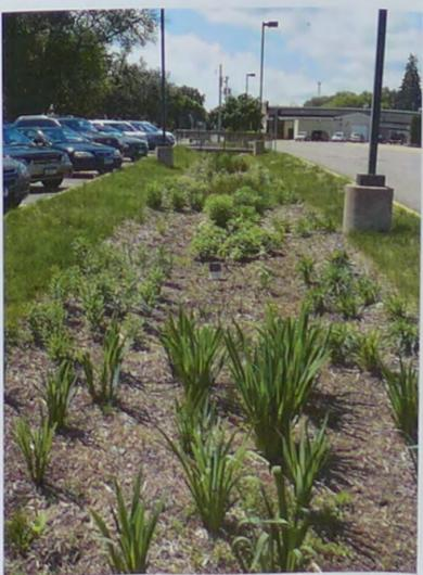
An infiltration swale is a long and narrow strip of land that infiltrates stormwater runoff from rain events into the ground, instead of "running off" into, and polluting surface waters
