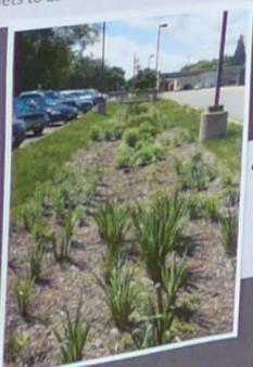
An infiltration swale is a long and narrow strip of land that infiltrates stormwater runoff from rain events into the ground, instead of "running off" into, and polluting surface waters
