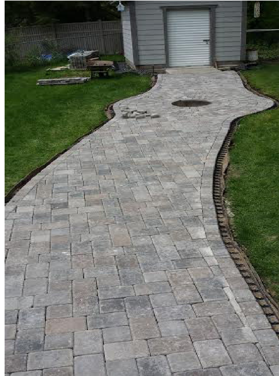
A pervious walkway installed in Vadnais Heights thanks to a Landscape 1 grant
